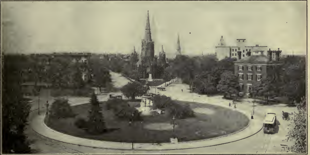
THOMAS CIRCLE, SHOWING THE RADIATING STREET SYSTEM
